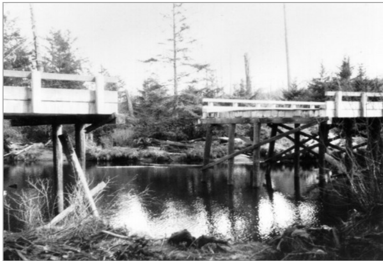
Bridge collapse on State Route 109 over Joe Creek in Grays Harbor County (Credit: U.S. Army Corps of Engineers)
