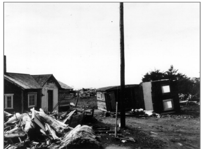
House torn apart from tsunami debris in Pacific Beach, Grays Harbor County (Credit: U.S. Army Corps of Engineers)
