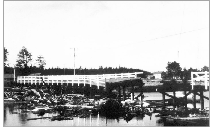
Bridge collapse after the tsunami debris came down the Copalis River (Credit: U.S. Army Corps of Engineers)
